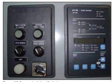
Figure 35.Bypass Isolation Switch.
